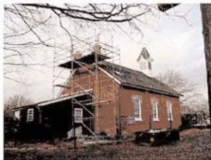
The schoolhouse was a construction site throughout most of the Fall.
