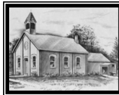
About 1920 with the second classroom at the back
